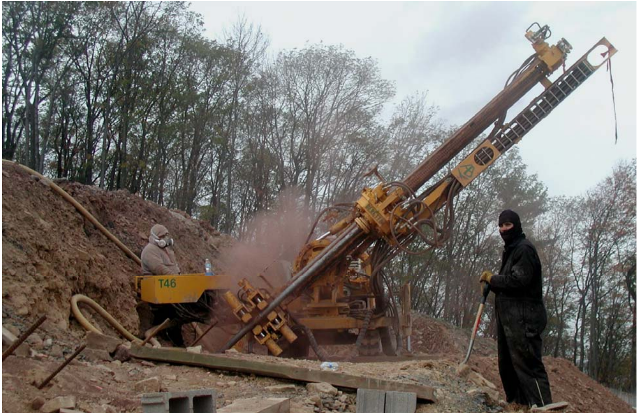
- Micropiles – Soil stabilization
