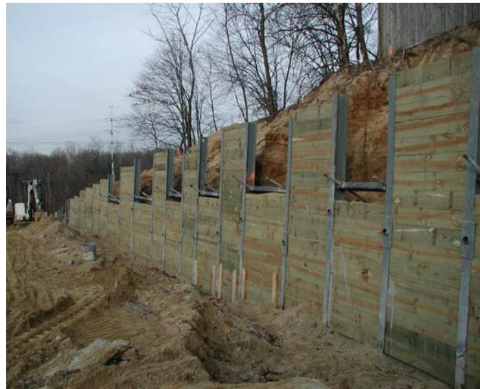
Micropiles – Tiebacks installation – Retention Wall
