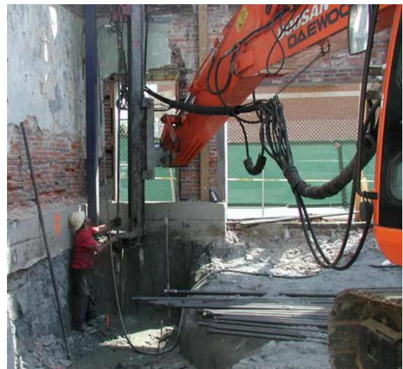
-Micropiles – New Foundation
